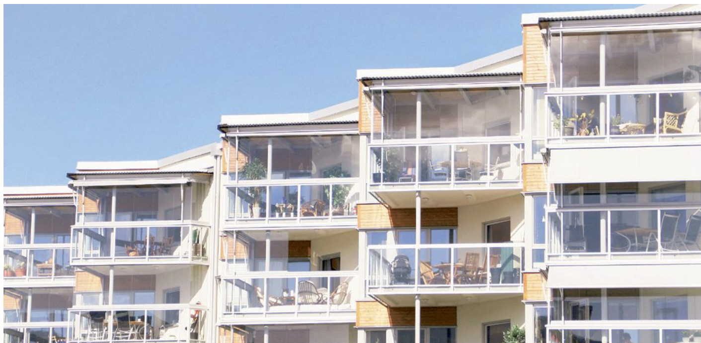
Landlord sub-metering offers clear cost-saving opportunities for the tenants, at the same time as it benefits the environment.
