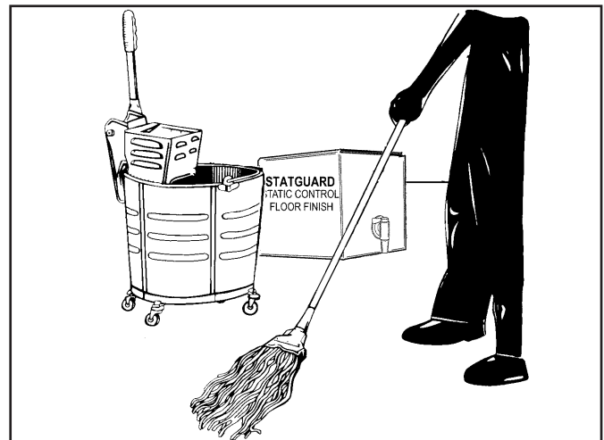
Figure 4. Applying floor finish.
